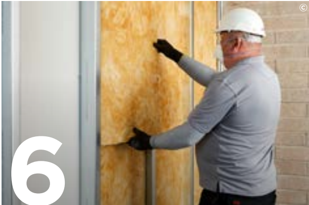
6 Add appropriate Isover insulation within the cavity.
