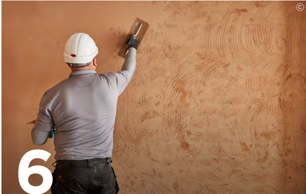
Allow the Thistle Undercoat Plaster to set. Apply Thistle Finish Plaster with firm pressure, build out to the required thickness in two applications and trowel to a smooth matt finish. It may be necessary to control the suction with Thistle GypPrime. Good site practice should be followed, as outlined in BS EN 13914-2, Design considerations and essential principles for internal plastering.
