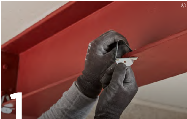
For three-sided protection to steel columns or beams, friction-fit Gypframe GL10 GypLyner Steel Framing Clips onto the column / beam flanges at 800mm centres.
