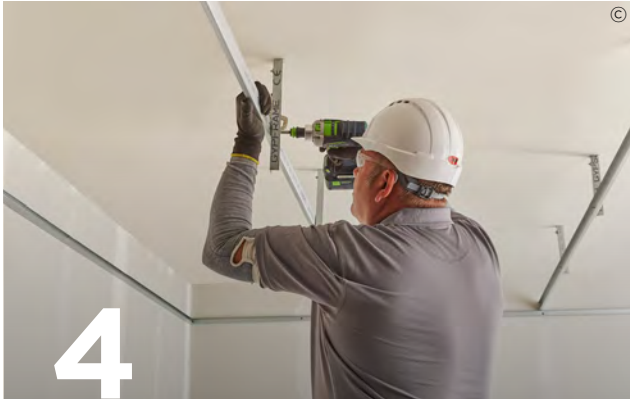
4 Position Gypframe MF7 Primary Support Channels then use British Gypsum Wafer Head Jack-Point screws to fix the hangers to the side of these channels. Use two screws per hanger.
