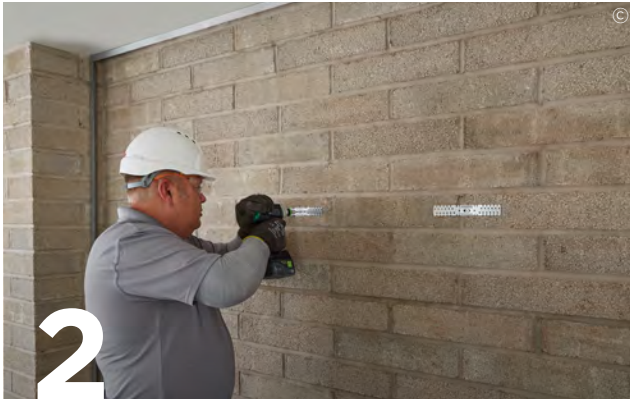
2 Mark vertical lines on the wall at 600mm intervals to indicate Gypframe GL2 or GL9 Bracket fixing centres. Mark horizontal lines at 800mm centres to determine individual bracket positions. Suitably fix Gypframe GL2 or GL9 Brackets into position. Gypframe GL2 or GL9 Brackets should be fixed with Gypframe GL11 GypLyner Anchor.
