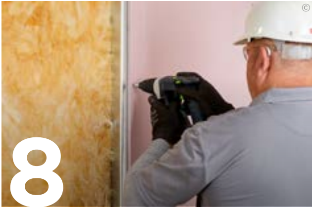
8 Use British Gypsum Jackpoint Drywall Screws to fix Gyproc plasterboards or Glasroc specialist boards to the SFS framework.
