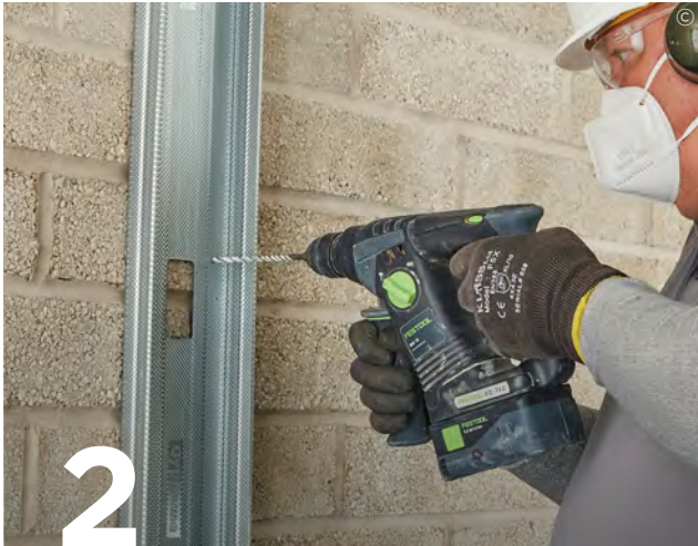
Fix Gypframe 'C' Studs at maximum 600mm centres to abutments and openings using suitable fixings.
