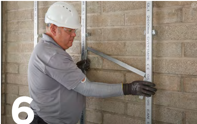
6 Construct door and window openings with Gypframe GL8 cut and bent to form the head of the opening and fix to the side of the channel using two British Gypsum Wafer Head Drywall Screws
