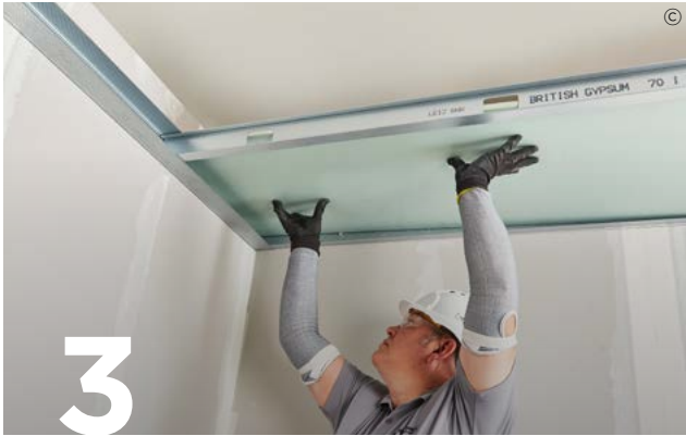
3 Friction fit Gypframe 'I' Studs or Gypframe Tabbed 'I' Studs into the channels at 600mm required centres. Fit Gyproc CoreBoard or 20mm Glasroc F FireCase between the studs on the shaft side.
