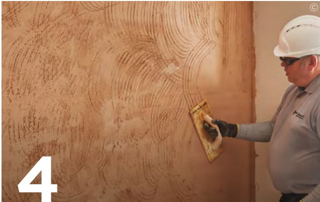
Rule the final coat to an even surface and lightly scratch to form a key.
