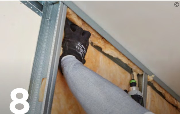
Add Isover Acoustic Partition Roll (APR 1200) insulation to the partition cavity for optimal acoustic performance.
