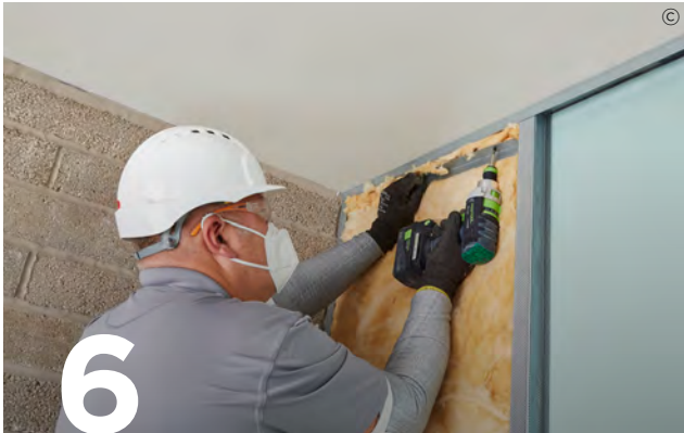
Add Isover Acoustic Partition Roll (APR 1200) insulation to the partition cavity for optimal acoustic and thermal performance.
