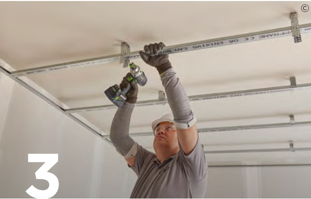
3 Position Gypframe GL1 Lining Channels into the perimeter track and between each leg of the Gypframe GL2, GL9 or GL12 Brackets. Use British Gypsum Wafer Head Drywall Screws to screw-fix the bracket to the Gypframe GL1 Lining Channels.
