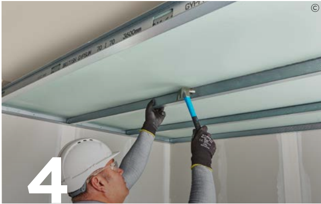
4 Use appropriate Gypframe Retaining Channels to hold boards in place.
