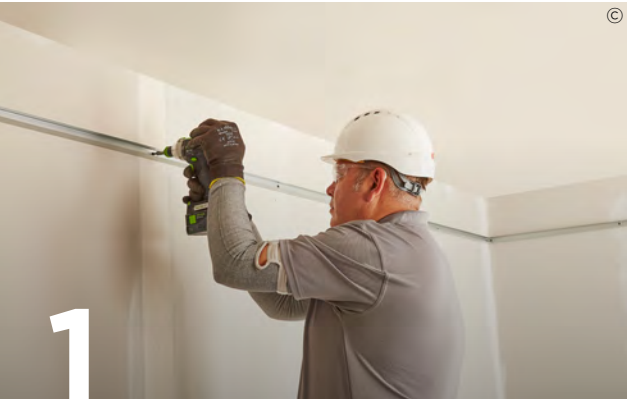
1 Fix Gypframe MF6 Perimeter Channels to the perimeter walls at 600mm centres.
