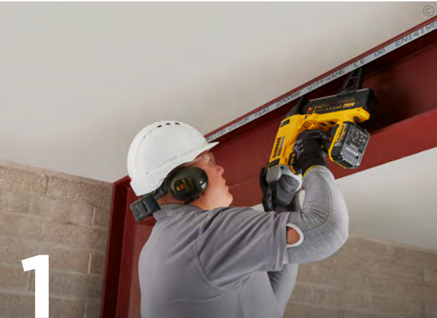
For two or three-sided protection to steel beams or columns, secure Gypframe FEA1 Steel Angles to both sides of the wall / soffit flange using appropriate fixings.
