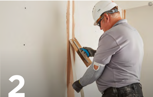
Where there is an increased risk of cracking, or where gaps exceed 3mm, the gaps are reinforced with Gyproc Joint Tape bedded in Thistle plaster. In other situations, plasterboard joints can be reinforced with Thistle ProTape FT50 or FT100 glass fibre mesh tape.
