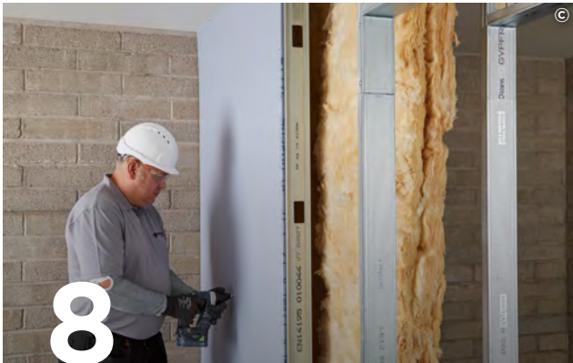
Use British Gypsum Jack-Point Screws to fix Gyproc plasterboards to the Gypframe framework.
