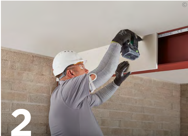
Cut Glasroc F FireCase boards to width and use Glasroc F FireCase Screws to fix to the Gypframe FEA1 Steel Angles.
