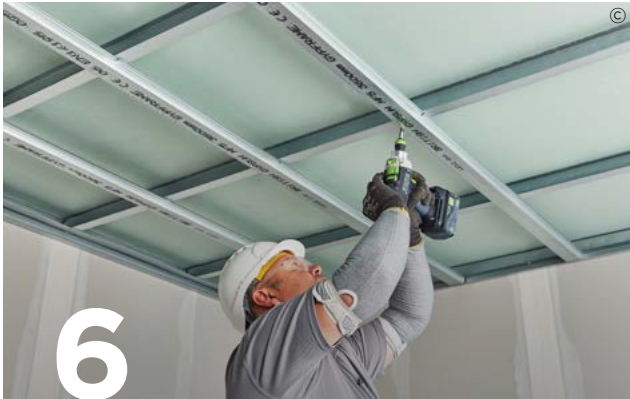
6 Run and fix Gypframe MF5 Ceiling Sections perpendicular to 'I' Studs using appropriate fixings.
