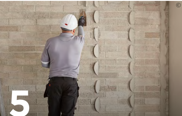
5 If using Gyproc DriWall Adhesive, apply methodically in a specific dab pattern to the appropriate background, ensuring 20% coverage is obtained.
