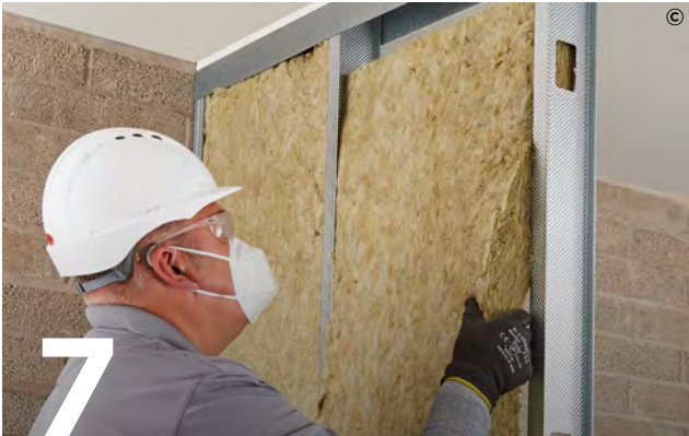
7 Stone mineral wool (by others) may be required as part of the partition installation, particularly for situations requiring enhanced fire resistance.
