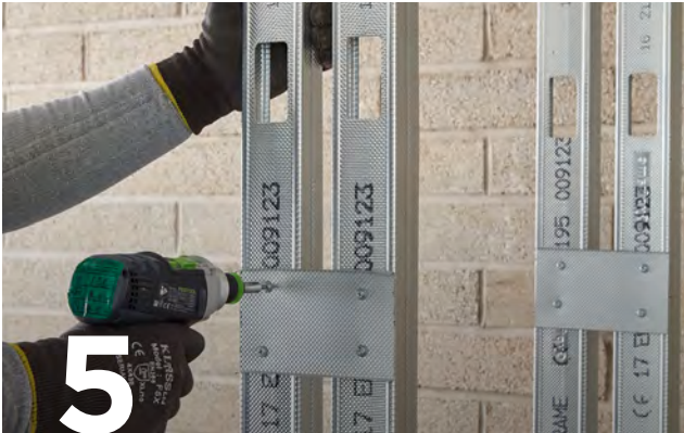
Brace the two frameworks are with a Gypframe 99 FC 50 Fixing Channel attached to the Gypframe 'C' Studs at 1200 centres. Use two British Gypsum Wafer Head Drywall Screws per junction.
