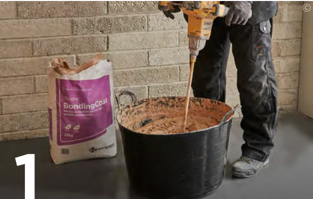
Mix Thistle plasters by adding to clean water and using clean mixing equipment. Avoid contamination from previous mixes as this can adversely affect the setting time and strength.
