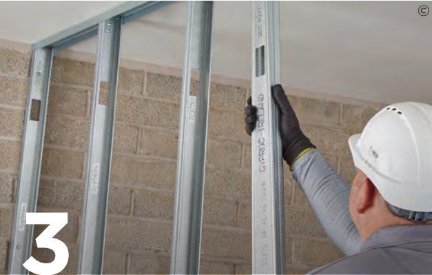
Friction fit Gypframe 'C' studs into the appropriate Gypframe Channels at required centres.
