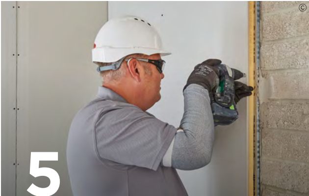
5 Use British Gypsum Drywall Screws to fix Gyproc plasterboards to the Gypframe MF10 Channel. Ensure correct length of screw is used to prevent thermal bridging.
