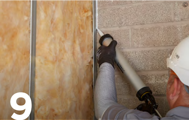
Use Gyproc Sealant to seal the perimeter of the partition except on the side where Gypframe RB1 Resilient Bars are to be installed. Where Gypframe RB1 Resilient Bars are to be installed, the Gyproc Sealant is applied to the perimeter of the first layer of board.
