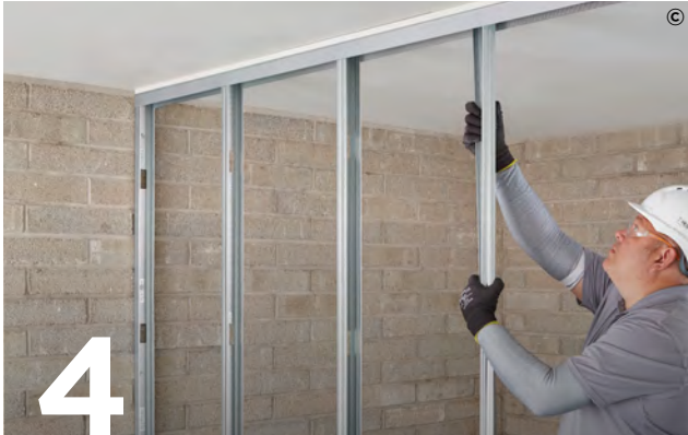
4 Friction fit Gypframe 'C' or 'I' studs into the Gypframe Floor & Ceiling Channels at required centres.
