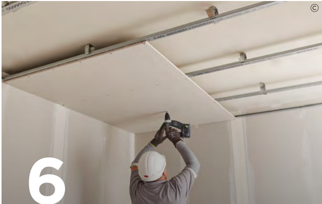
6 Suitably fix boards to form one or two layer linings as specified using appropriate fixing at 90 degrees to the Gypframe GL1 Lining Channels and Gypframe GL8 track. Important point - Use British Gypsum Drywall Screws to fix GL6 Timber Connectors to the side of the joists. The connectors must be aligned accurately and level as they cannot be adjusted once Gypframe GL1 Lining Channel is engaged into a row of timber connectors and twisted into position. See specific detail for more information.
