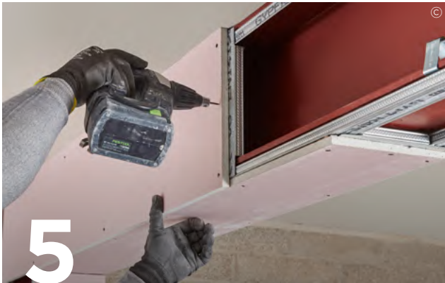
For single layer beam encasements board-end joints are backed using vertical noggings formed from an appropriate Gypframe component: Gypframe GL1 Lining Channel, Gypframe GFS1 Fixing Strap or Gypframe GFT1 Fixing 'T'.
