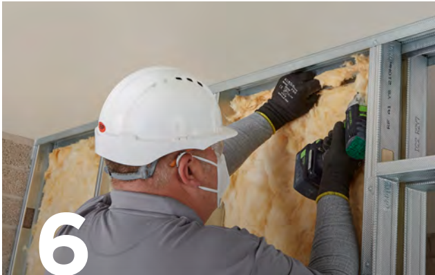
Add insulation to the partition cavity for optimal acoustic and thermal performance.
