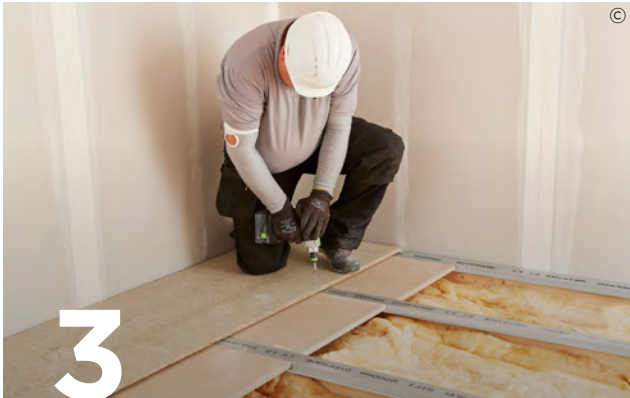
3 Lay flooring across the Gypframe SIF Floor Channels. Use Gypframe SIF5 Floor Screws to fix through the Gyproc Plank to the channel flange on one side only.
