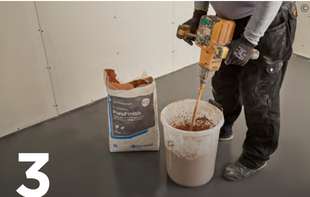
Thistle plasters should be mixed by adding to clean water and using clean mixing equipment. Contamination from previous mixes must be avoided as this can adversely affect the setting time and strength.
