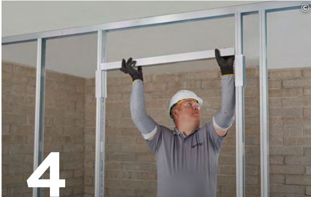
4 Construct door openings to the Heavy and Severe rating door detail.
