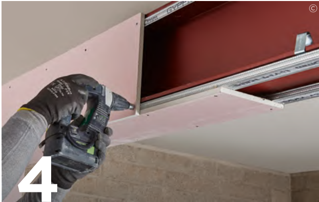
Use British Gypsum Drywall Screws to fix cut boards to all framing members.
