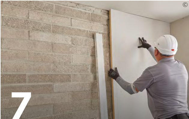
7 Offer up boards and tap into position. Be careful to avoid creating wave and hollows.
