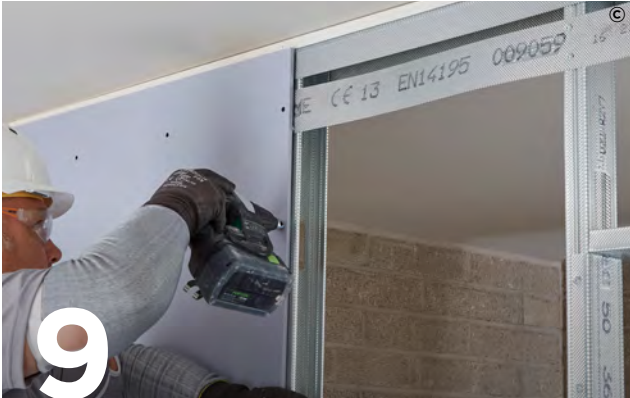
9 Use British Gypsum Drywall Screws to fix Gyproc plasterboards or Glasroc specialist boards to Gypframe framework.
