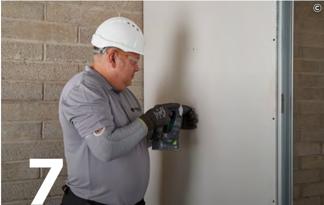
7 Use British Gypsum Drywall Screws to fix Gyproc DuraLine (and Gyproc SoundBloc inner layer if required) plasterboards to the Gypframe framework.
