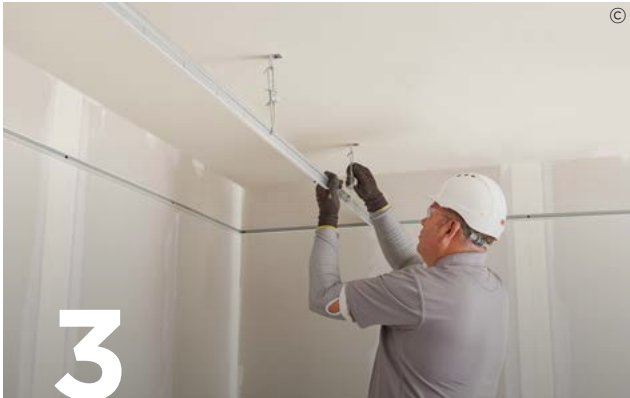
3 Use CasoLine Quick-Lock Grid Hangers to suspend the CasoLine Quick-Lock Grid Main Tee 24/38 or 15/38 Main Tee.
