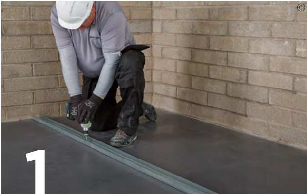
Suitably fix the appropriate Gypframe Floor & Ceiling Channels at the required centres to the floor and soffit.
