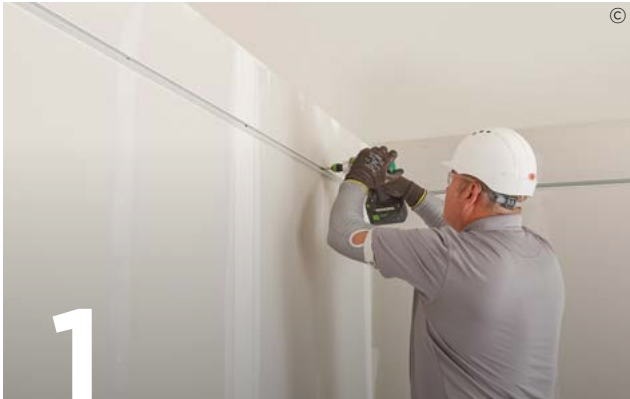
1 Measure and mark the required ceiling height. Fix the CasoLine Quick-Lock Grid Wall Angle WA02 or WA03 around the perimeter of the ceiling area.
