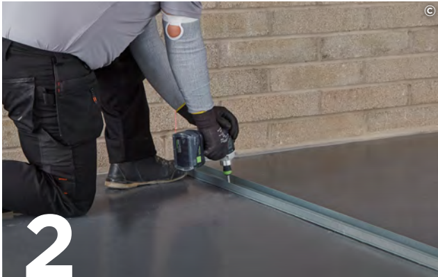
2 Suitably fix the appropriate Gypframe Floor & Ceiling Channels at the required centres to the floor and soffit. Important note - for channels 72mm and below a single row of fixings are used. For anything above 72mm two rows of 600mm fixings staggered by 300mm are used.
