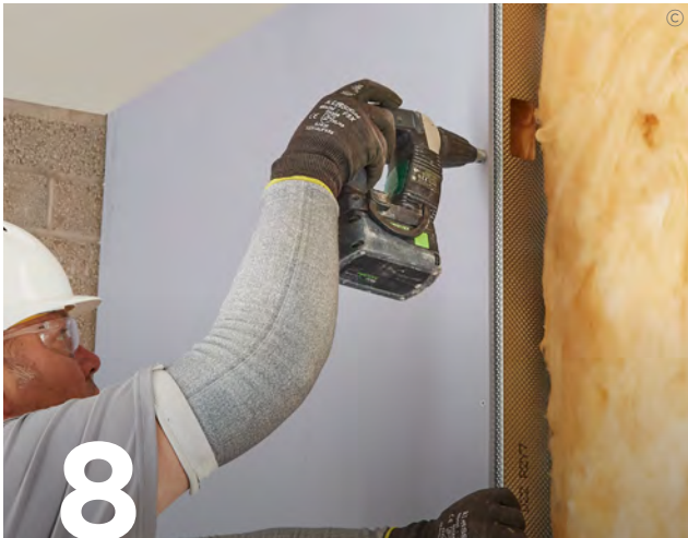
Use British Gypsum Jack-Point Screws to fix Gyproc SoundBloc plasterboards to alternate Gypframe 'I' Studs and other framing members.
