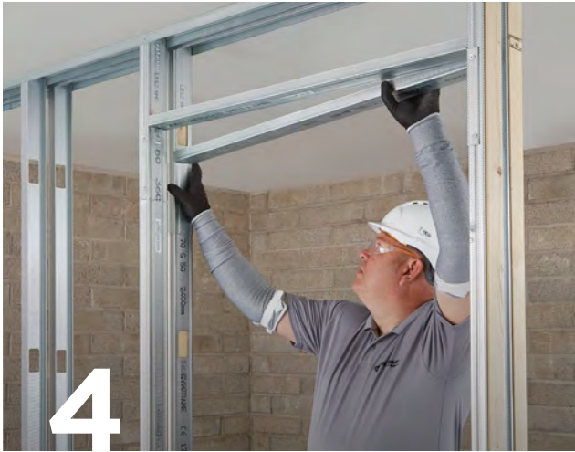
Construct door openings to suit Severe Door Duty Rating detail.
