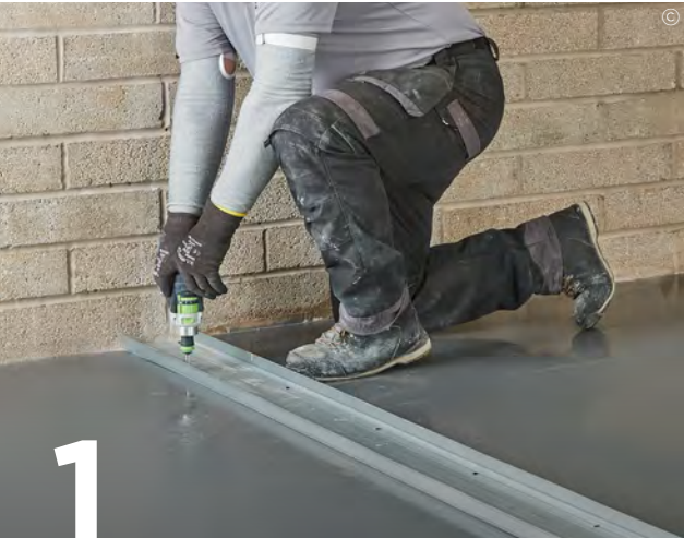
Suitably fix the appropriate Gypframe Floor & Ceiling Channels at the required centres to the floor and soffit.
