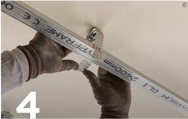
4 Bend the protruding legs of each bracket to sit back from the channel face. Important point - Gypframe GL1 Lining Channel sections are extended using Gypframe GL3 Channel Connectors.
