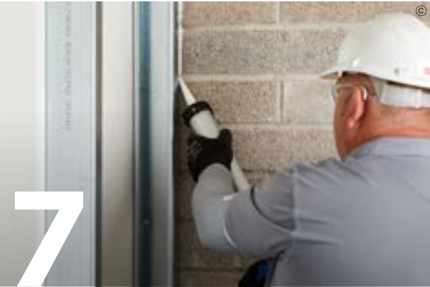
7 Use Gyproc Sealant to seal the perimeter.
