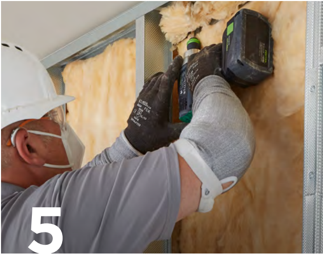
Add Isover Acoustic Partition Roll (APR 1200) insulation to the partition cavity for optimal acoustic and thermal performance.
