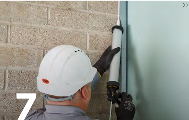
Use Gyproc Sealant to seal the frame perimeter.
