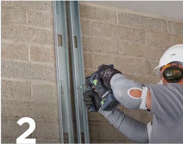
Fix Gypframe 'C' Studs to abutments and openings in two rows using suitable fixings.
