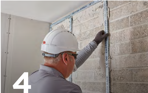
4 Position Gypframe MF10 Channels onto the adhesive dabs and tap into position. Locate horizontal channels at the head and base using the same method.
