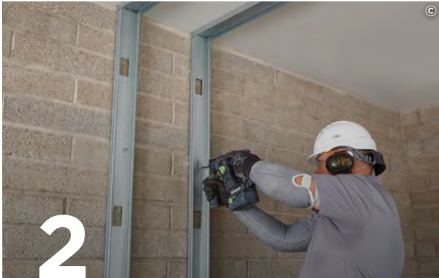
Fix Gypframe 92 S 10 'C' Studs at abutments and door openings in two rows using suitable fixings.
