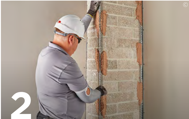
Fix a Thistle Plaster Angle Bead or Thistle Plaster Stop Bead to the background by embedding in the undercoat plaster. Where Thistle BondingCoat undercoat plaster is to be applied to plasterboard, reinforce the board joints with Gyproc Joint Tape bedded in Thistle plaster.
