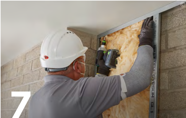
7 Add Isover Acoustic Partition Roll (APR 1200) insulation to the partition cavity for optimal acoustic and thermal performance.
