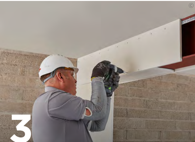
Where Glasroc F FireCase boards abut fix together with Glasroc F FireCase Screws. For four-sided protection to steel columns, Glasroc F FireCase boards are positioned and fixed board to board using Glasroc F FireCase Screws. Ensure that board-to-board edge fixings are secured into the centre of the Glasroc F FireCase soffit board.
