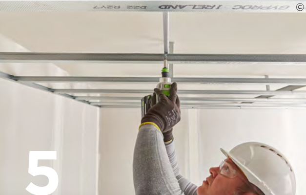
5 Use British Gypsum Wafer Head Jack-Point Screws to fix Gypframe MF5 Ceiling Sections to the underside of the Gypframe MF7 Primary support at required centres.
