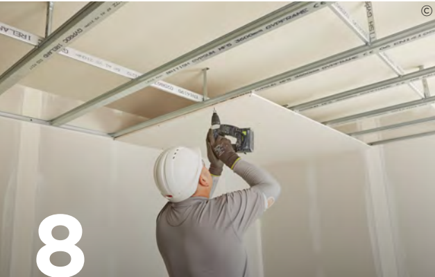
8 Use the appropriate fixing to fix Gyproc plasterboards, Glasroc specialist boards, Gyptone boards or Rigitone boards to the Gypframe MF5 Ceiling Sections and Gypframe MF6 Perimeter Channels.
