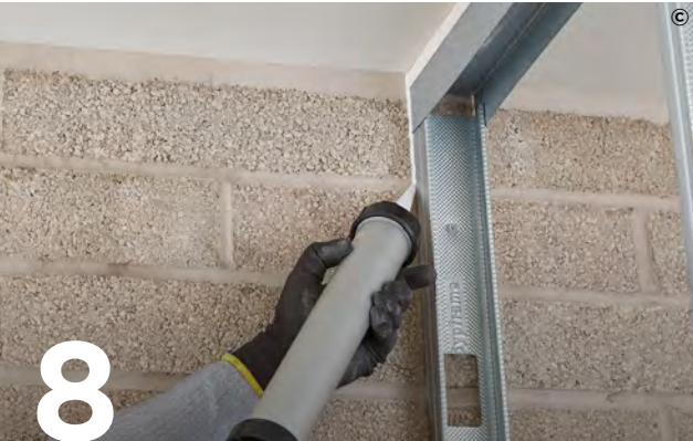
8 Use Gyproc Sealant to seal the perimeter of the partition.
