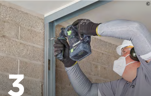
3 Fix Gypframe 'C' Studs to abutments and openings using suitable fixings.
