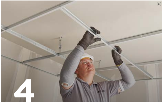
4 Install 600mm and/or 1200mm CasoLine Quick-Lock Grid 24/38 Cross Tee or 15/38mm Cross Tee as required.
