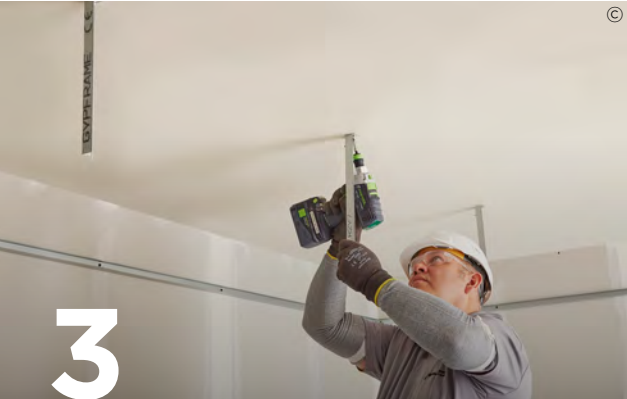
3 Suitably fix these hangers to the soffit at the required centres.
