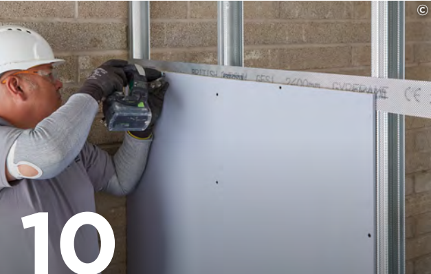
10 Important note: For single and double outer layer horizontal board joints use a Gypframe GFS1 Fixing Strap to maintain fixing centres
