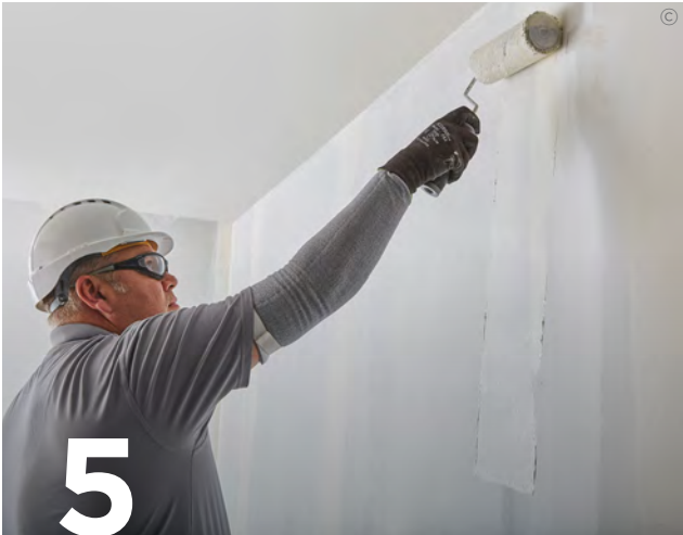
Gyproc Drywall Primer or Gyproc Drywall Sealer is applied to the entire board surface and jointed areas, to control suction and prepare the lining for final decorative treatment.
