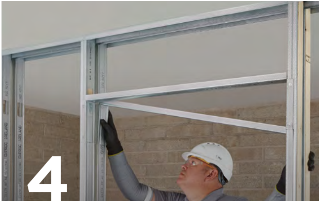
Construct door openings to the Severe Duty rating door detail.
