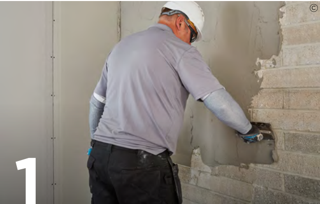
1 Apply Gyproc SoundCoat Plus in a continuous 6mm coat to the entire surface of the external or separating walls for optimum air tightness and acoustics. Allow Gyproc SoundCoat Plus to set before applying of DriLyner Dab using Gyproc DriWall Adhesive.
