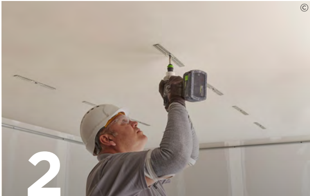
2 Suitably fix Gypframe GL2, GL9 or GL12 Brackets as required to the soffit at the required centres.
