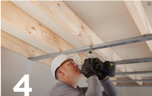
4 Use British Gypsum Drywall Screws to install Gypframe RB1 Resilient Bars to the underside of the joists.
