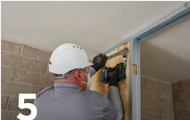
Add Isover Steel Infill Batt or Isover Acoustic Partition Roll (APR 1200) to the partition cavity for optimal acoustic and thermal performance.
