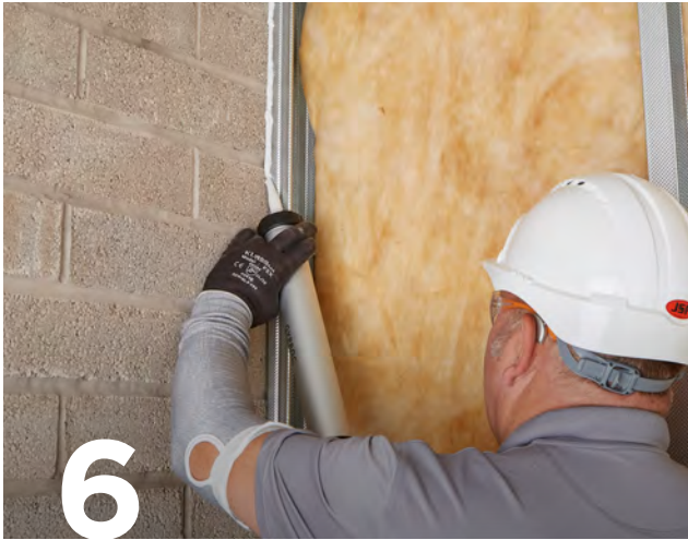
Use Gyproc Sealant to seal the perimeter of the partition.
