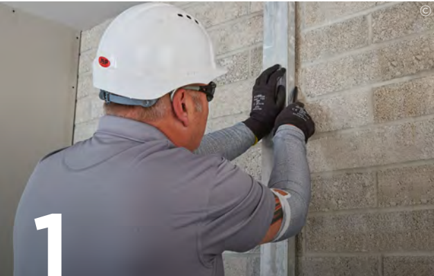
1 Mark the board edge positions on the wall or plasterboard to aid the correct and accurate application of the Gyproc DriWall Adhesive.
