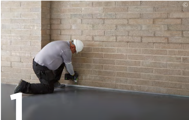
1 Suitably fix Gypframe GL8 Track to the perimeter walls at the required centres. Ensure the large lip faces internally.
