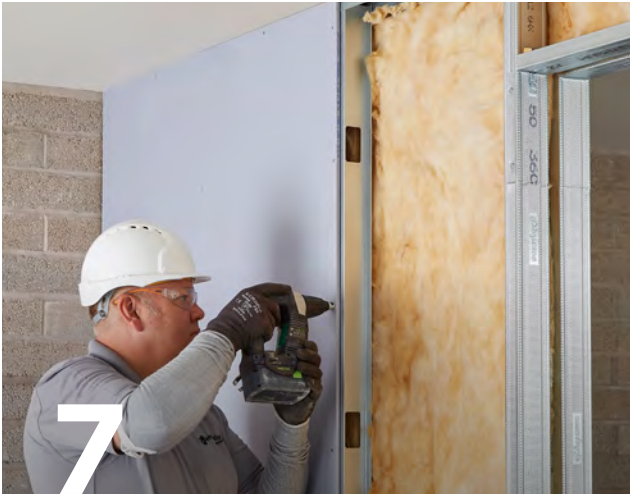
Use British Gypsum Drywall Screws and British Gypsum Jack-Point Screws to fix Gyproc plasterboards to the Gypframe framework.
