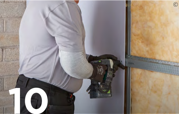
Use British Gypsum Drywall Screws to fix Gyproc plasterboards to the Gypframe RB1 Resilient Bars, with all joints staggered.
