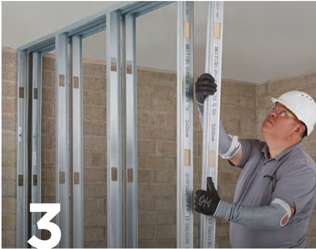
Friction fit Gypframe 'I' Studs into the appropriate Gypframe Floor & Ceiling Channels at the required centres.
