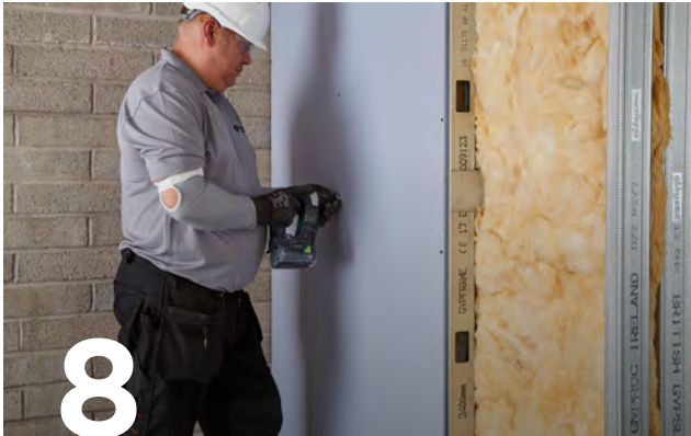
Use British Gypsum Drywall Screws to fix Gyproc plasterboards to the Gypframe framework.
