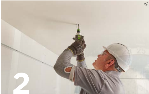
2 Mark the ceiling at the required centres for the suspension points and fasten the Gypframe MF12 Soffit Cleats to the soffit.
