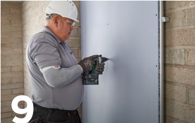
9 Use British Gypsum Drywall Screws to fix Gyproc plasterboards or Gyproc ThermoLine to all framing members.
