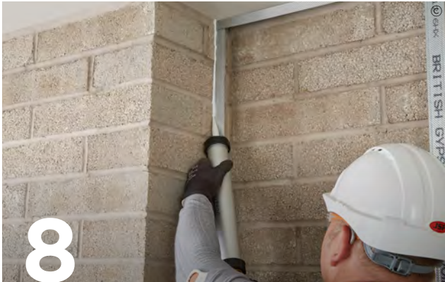
8 Use Gyproc Sealant to seal the perimeter of the lining.
