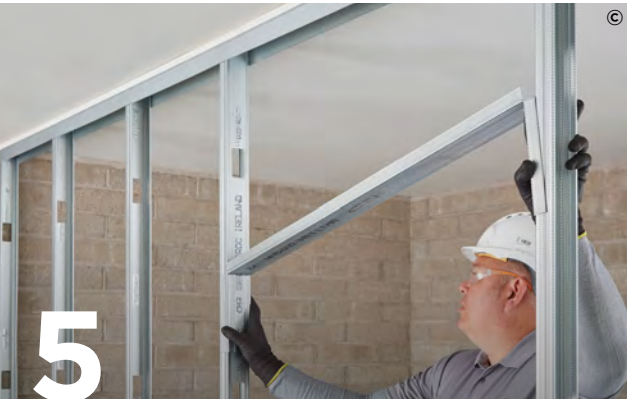
5 Construct door openings to meet the partitions' duty rating.
