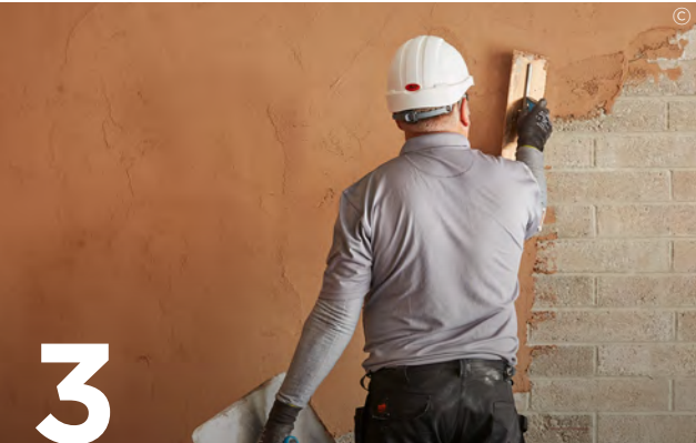
Select the correct Thistle plaster to suit the background suction and surface texture. Apply the plaster in maximum 8mm coats. Allow each coat to set before applying the next.
