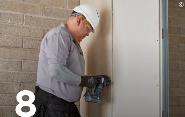
8 For an even more robust solution use Rigidur Screws to fix Rigidur H as the outer layer to all Gypframe framing members.
