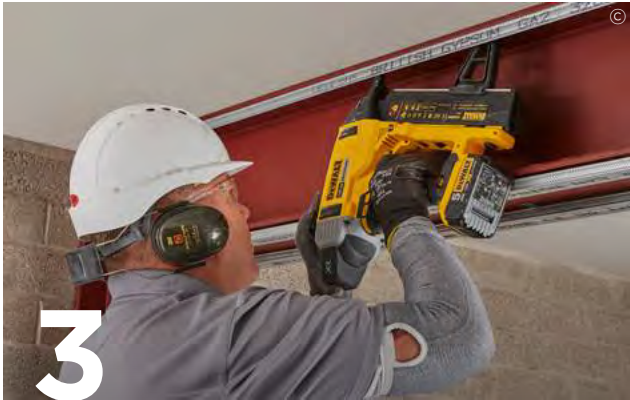
For two or three-sided beams or columns, use appropriate fixings to secure Gypframe GA2 Steel Angles to both sides of the wall / soffit flange.
