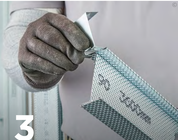
Insert Gypframe Spacer Clips to the top and bottom of the studs. Use Gypframe SC1 when using Gypframe 60 I 70 'I' Studs. Use Gypframe SC2 Spacer Clips when using Gypframe 92 I 90 'I' Studs.
