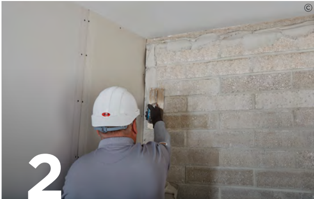
2 Apply a continuous fillet / ribbon of Gyproc DriWall Adhesive to the wall perimeter and around all services and openings. This is particularly important if the lining is designed to act as an air barrier to achieve building airtightness.
