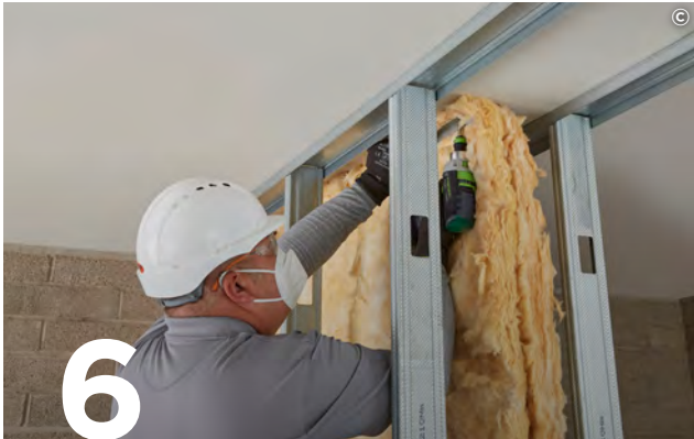
Add Isover Cladding Roll 40 insulation to the partition cavity for optimal acoustic and thermal performance.
