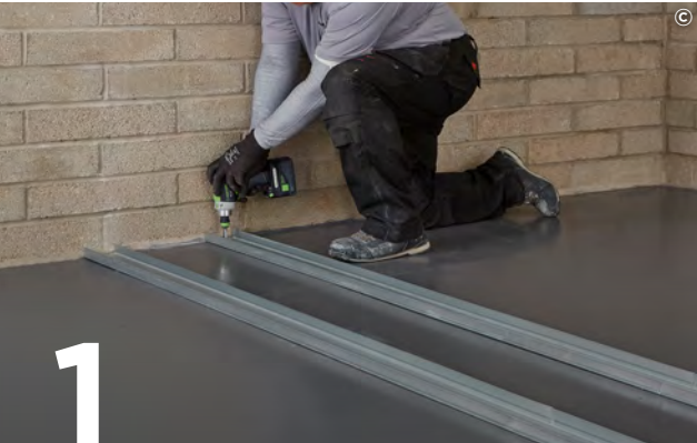
Suitably fix the appropriate Gypframe Floor & Ceiling Channels at the required centres to the floor and soffit. Important note – for channels 72mm and below a single row of fixings are used. For anything above 72mm two rows of 600mm fixings staggered by 300mm are used. For deflection heads see suitable details.
