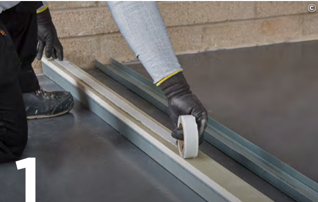
1 If a deflection head is required start by creating the dropped soffit, cut the appropriate depth and width of Gyproc plasterboard or Glasroc specialist board and attach to your head channel. Locate intumescent Gyproc FireStrip as per the detail.
