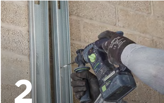
Fix Gypframe 'C' Studs at abutments and openings in two rows using suitable fixings.
