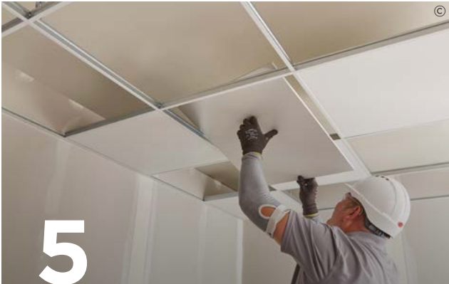
5 Lay the ceiling tiles into place. Important point - CasoLine Quick-Lock Grid is a self-squaring system, with the main tees and cross tees now in place the ceiling tiles should be easily laid into place. Important point - Ceiling tiles should be intermittently spaced around the CasoLine Quick-Lock Grid system to enable the frame to stay square.
