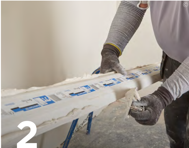
Profiles are cut to length using a fine-tooth saw and mitred using a suitable mitre block. Gyproc Cove Adhesive or Gyproc EasiFill is evenly applied to both surfaces that will be in contact with the wall and ceiling.
