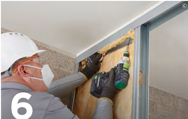
6 Add appropriate Isover insulation (Acoustic Partition Roll (1200) as shown) within the partition cavity to contribute to acoustic and thermal performance where required.
