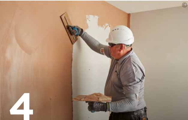
Thistle plaster is applied with firm pressure, built out to the required thickness in two applications and trowelled to a smooth matt finish. When applying ThistlePro FastSet Finish, a single mix for both first and second coat is recommended.
