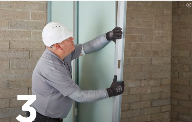
Friction fit Gypframe 'I' Studs or Gypframe Tabbed 'I' Studs into the channels at 600mm required centres. Fit Gyproc CoreBoard or 20mm Glasroc F FireCase between the studs on the shaft side.
