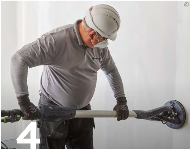
Once dried, the joint treatment is sanded as necessary to achieve a smooth surface.
