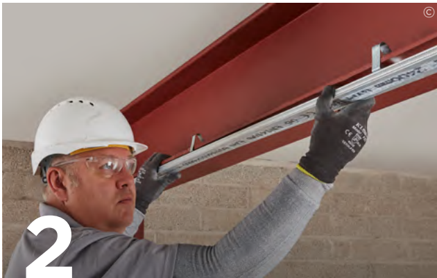
Locate Gypframe GL1 Lining Channels over the clips to form the steel framework.
