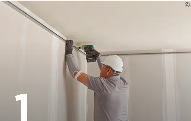
1 Suitably fix Gypframe GL8 Perimeter Channels to the perimeter walls at the required centres. Ensure the large lip is positioned at the bottom.
