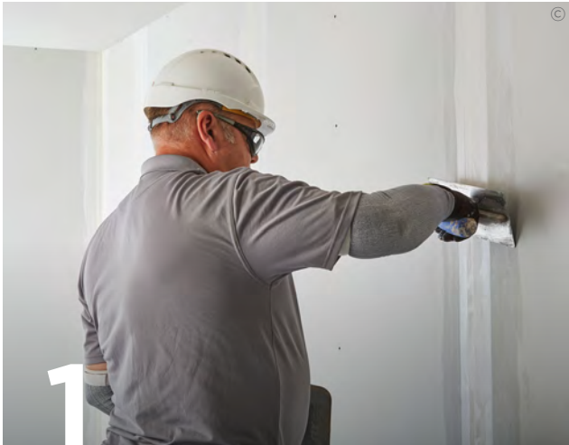
Gyproc Joint Tape is bedded into the appropriate Gyproc jointing compound to all board joints and internal corners.
