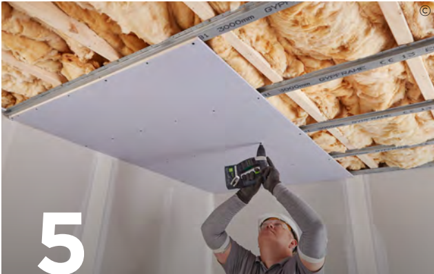
5 Lay 100mm Isover Spacesaver Ready-Cut between joists and rest on the Gypframe RB1 Resilient Bars. Use British Gypsum Drywall Screws to fix the specified ceiling board fixed to the Gypframe RB1 Resilient Bars.
