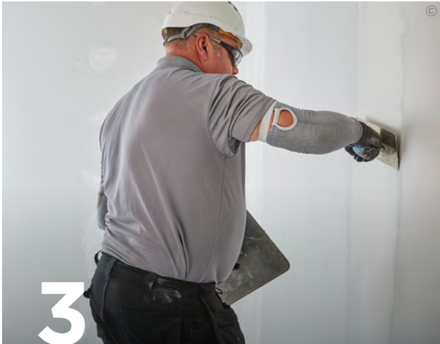
Two or three further applications of jointing compound are trowel applied, each feathered out beyond the previous application. An equal number of applications are made to spot screw heads.
