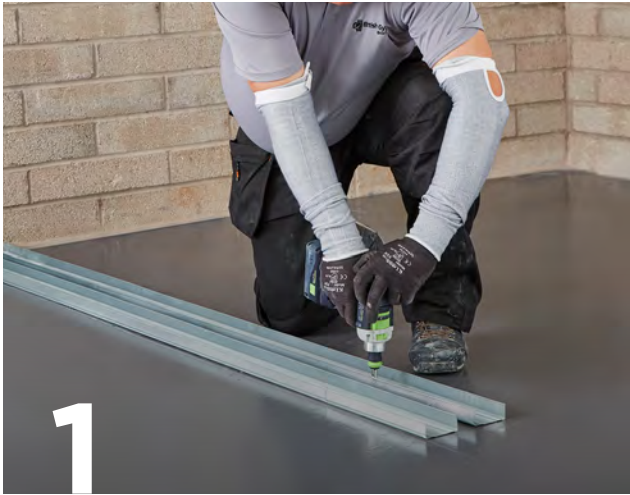
Suitably fix the appropriate Gypframe Floor & Ceiling Channels in two rows at the required centres to the floor and soffit.
